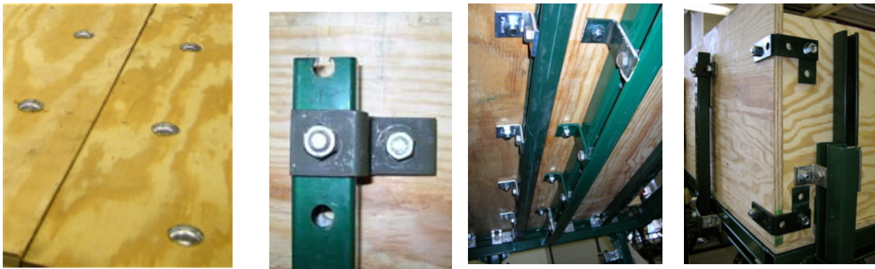
Figure 4: Typical UNISTRUT® connections and channel bolt use on plywood
