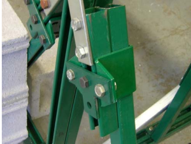
Figure 10.8: Unistrut 1001C connector Solution 2
