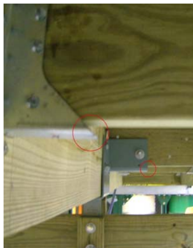
Figure 10.1: Diaphragms Requiring Bottom Shims
