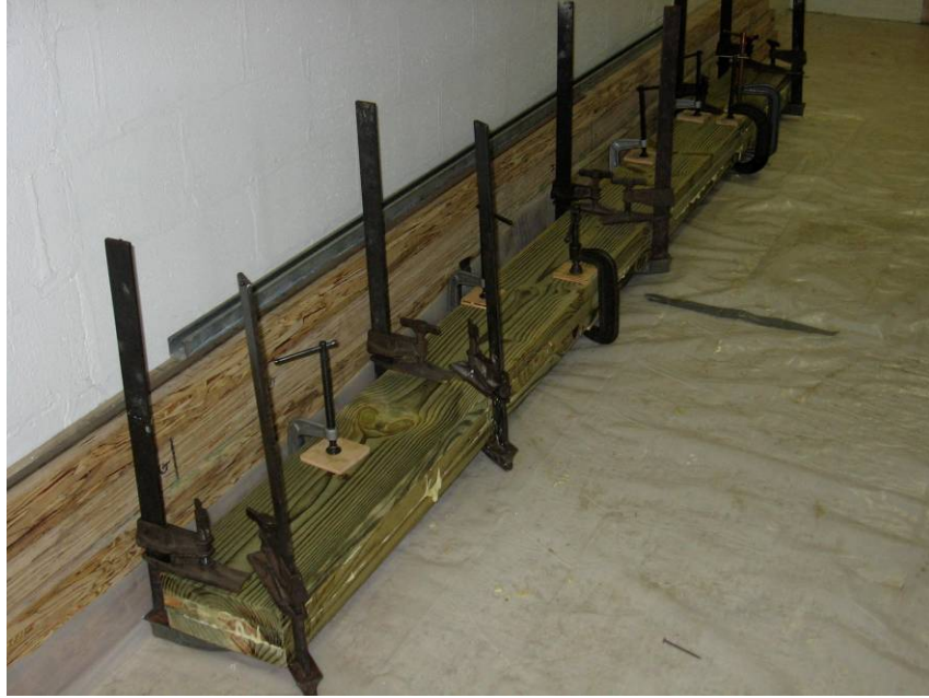
Figure 5.1: Fabrication of Built-Up Girders: Clamped after Gluing
