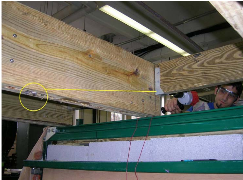
Figure 5.7: Wood Drill and Extender Going Through the entire 28" Hole
