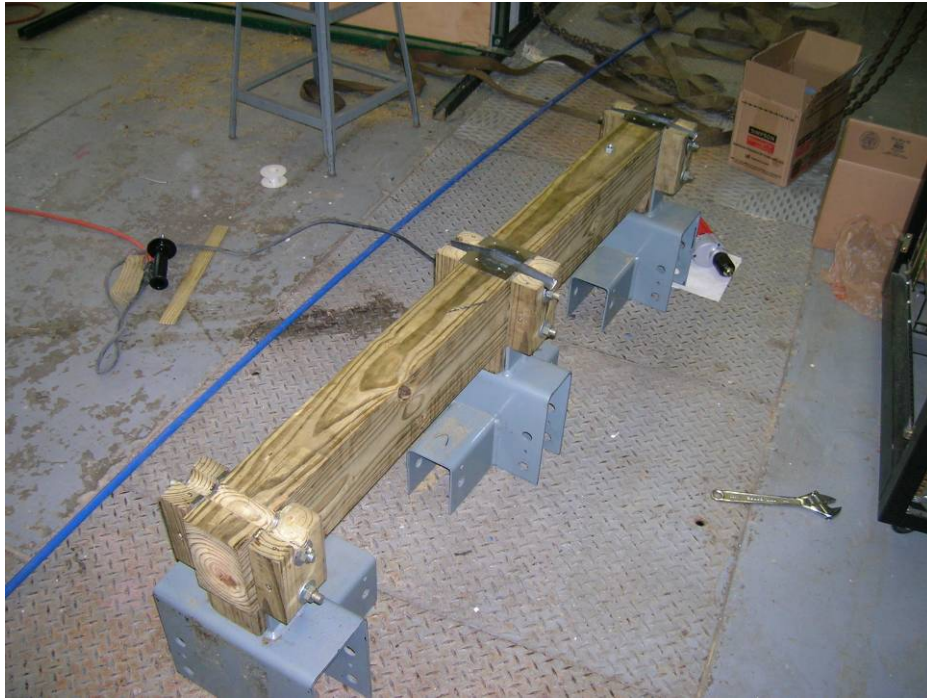
Figure 5.6: King Post Construction Showing Milled Grooves and Half-Pipes
