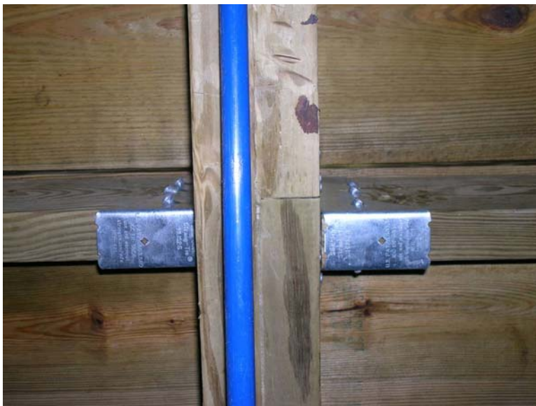
Figure 10.4: Quarter Point Diaphragms Staggering
