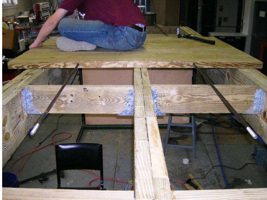
Figure 5.11: Deck Planks Being Pushed onto Deck Rods
