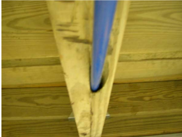
Figure 10.5: Cable Exiting Central Girder Slightly Off-Center
